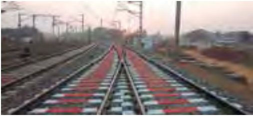
Kharagpur third line project, West Bengal.
