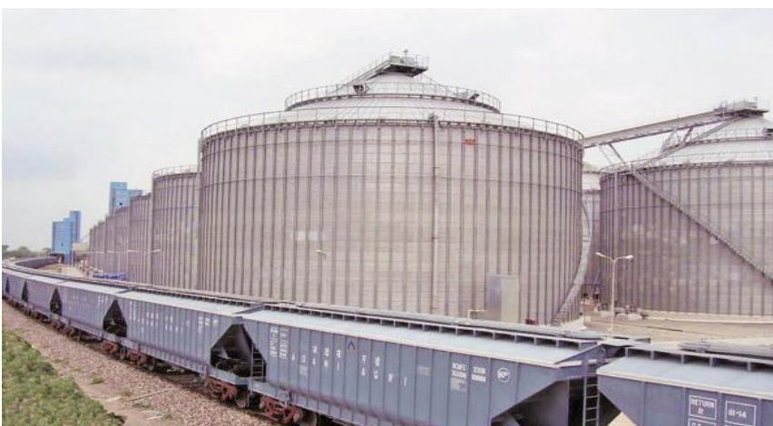
View of Food Grain Storage Silos
