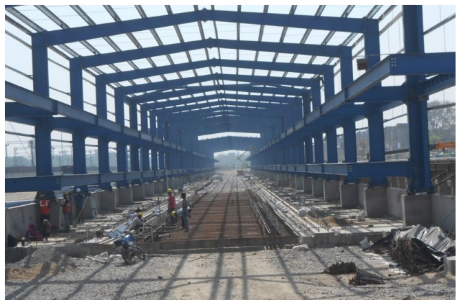
Kanpur MEMU Shed Project: Construction in progress at Inspection Shed
