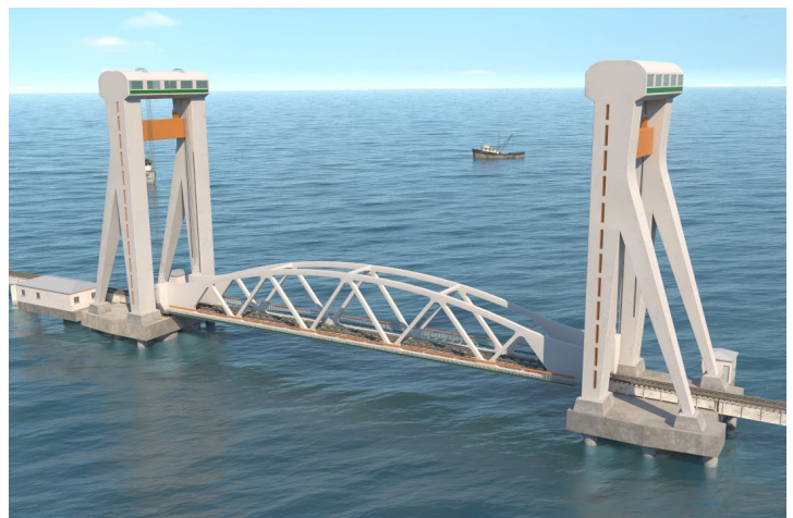
Vertical Single Lift Span
