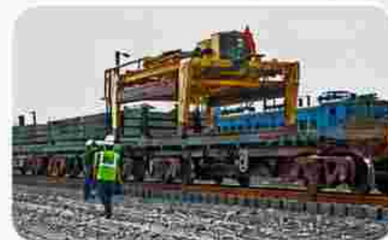
Dadri-Khurja section, Dedicated Freight Corridor
