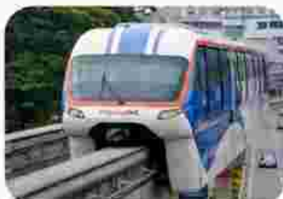
Safety Audit for Kuala Lumpur Monorail
