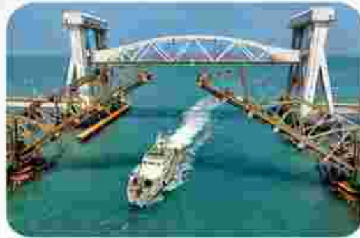
Pamban Bridge – Vertical Lift Sea Bridge
